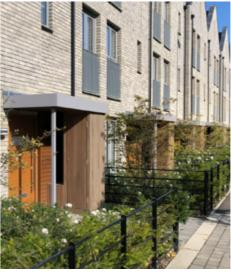
Fig 10.13 Examples of waste and recycling storage integrated into the porch of an individual dwelling
