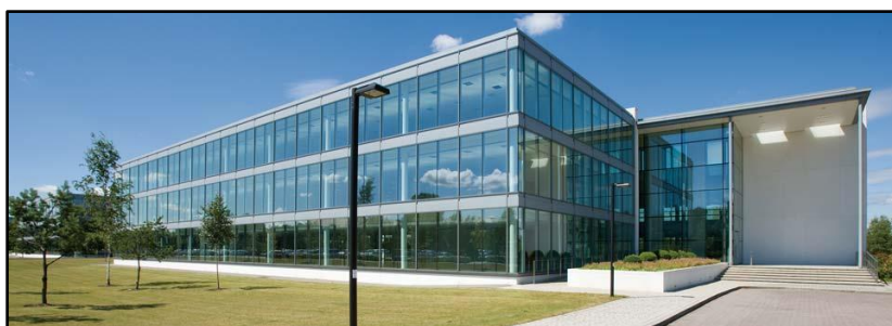
Figure 1 Modern A Grade office space at The Heights, Weybridge
