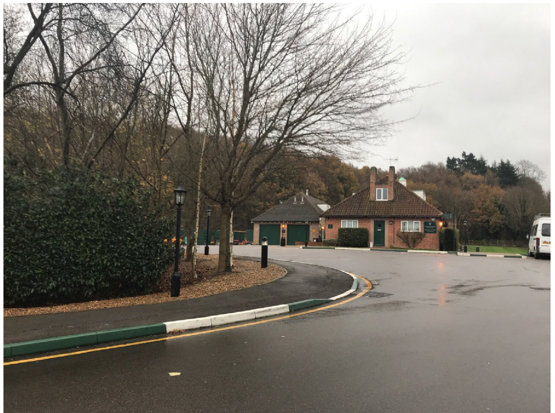
Photograph 2 Facing east towards sports pavilion in the centre of SA-62.
