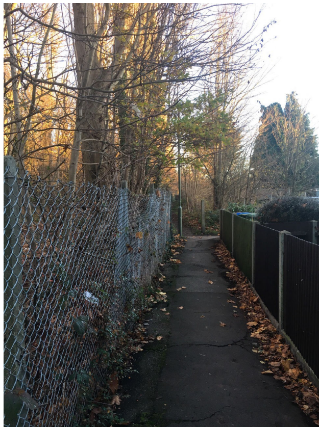
Photograph 2 View of southern boundary of SA-66, formed of tree line, fence and footpath, facing east.
