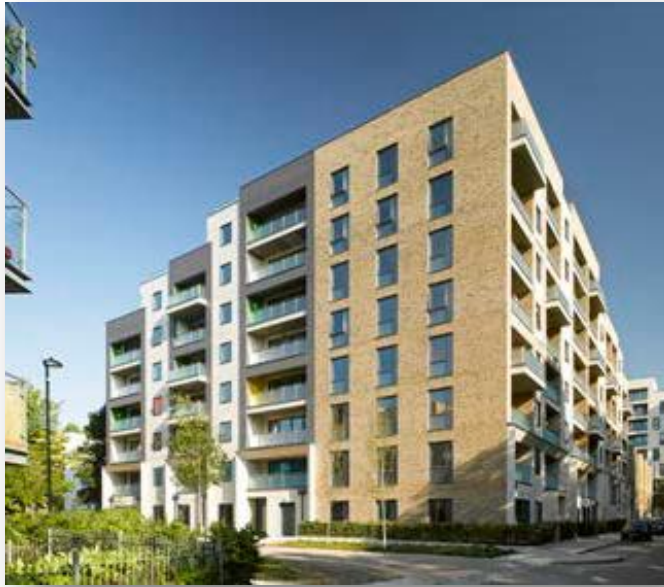
Figure 7: Image: South Action Phase 1, Architect: HTA Design LLP
