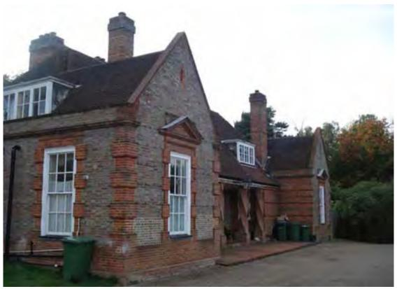
Fig. 35: The notable use of grey headers with red brick dressing to The Manse
