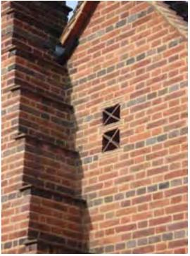
Fig. 36: String courses or banding of grey brick (note ventilation detail)
