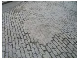
Fig.61 Poorly repaired cobble surface to the Wharf.
