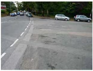
Fig.60 Patched and pot-holed tarmac surface at the entrance to the section of Manor Road leading to the river front.
