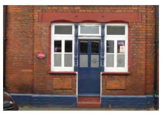
Fig.24 A detail of the George Inn – red brick in Flemish bond with terracotta detailing and rubbed brick panels.
