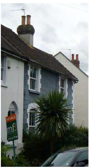
Fig.41 The notable use of what appears to be a stone for the walling of this house could be evidence of building materials being transported by river from further afield and of considerable local interest.
