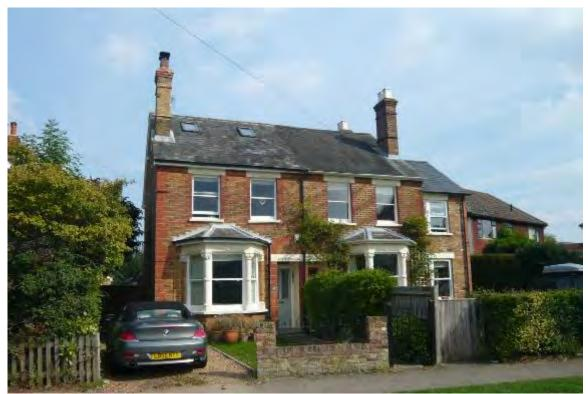
Figure 8: Mirrored plans and shared architectural features to semi-detached houses
