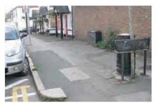
Figure 17 Poor quality paving surfaces, top end High Street
