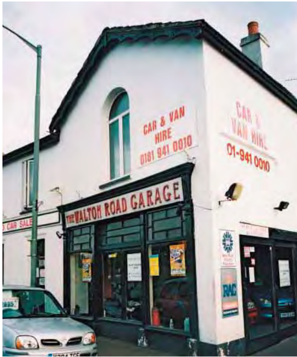
No.34 Walton Road. A surviving well detailed shopfront of c.1920.
