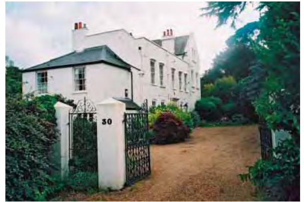
Green Arden - A grade II building which dates from the early 18th century.
