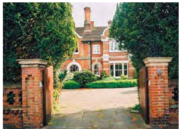
No.25 Matham Road a notable locally listed house.
