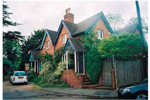
Architectural detailing is an important part of the area's special character (nos. 24 & 26 Spencer Road).
