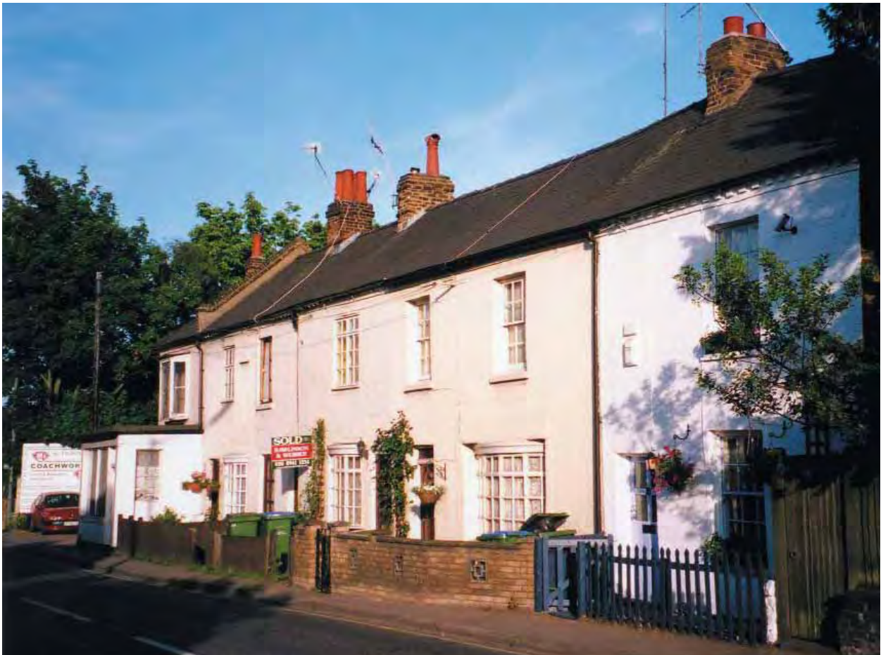
Late 18th century cottages on Walton Road.
