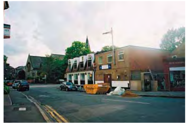
The gateway into St Mary's Road is marred by St Andrews Hall.
