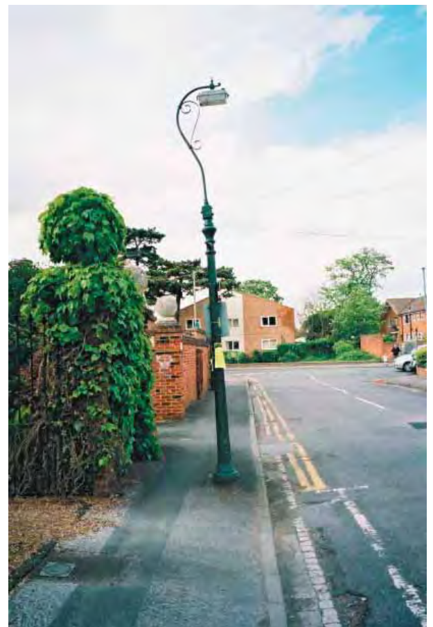
Lamp column, Matham Road
