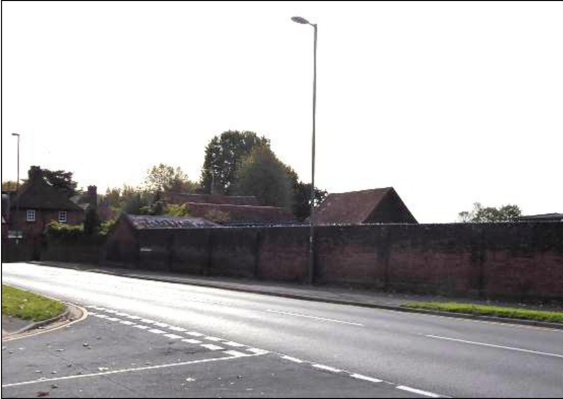
Figure 13: Pyports and its outbuildings and boundary wall to Downside Bridge Road
