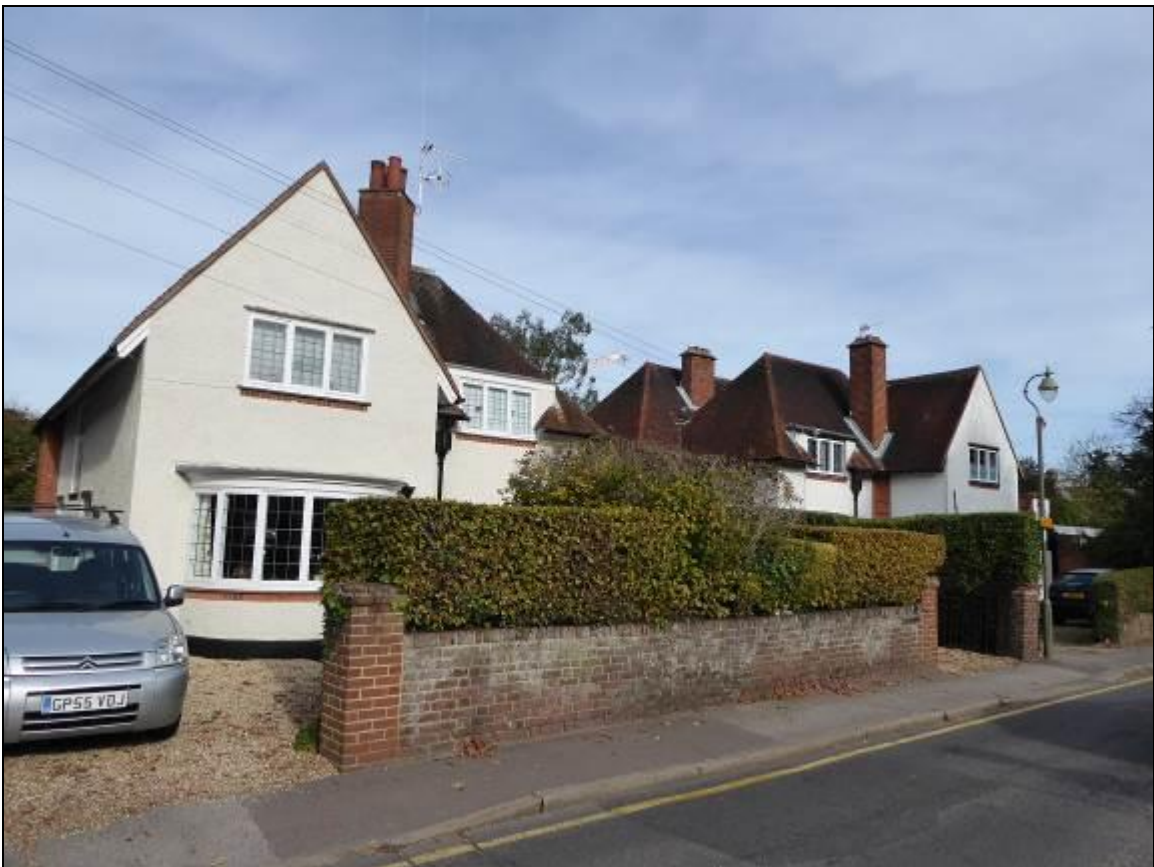
Figure 19: Nos. 12 and 14 Church Street designed by local architect Leonard Martin
