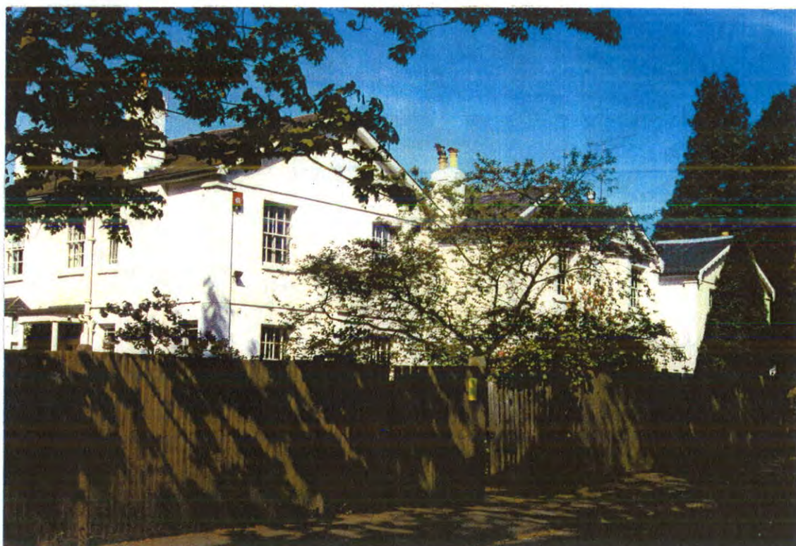
11. OAK TREE HOUSE, CHURCH VILLAS AND TRINITY COTTAGE, CHURCH ROAD
