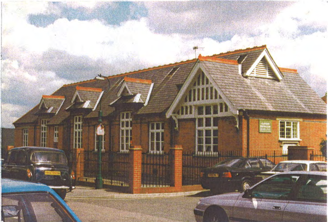
7. THE OLD SCHOOL BUILDING – ELM ROAD
