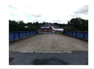
Looking across the bridge towards the Museum, the original concrete surface and kerbing remains although degrading in some areas
