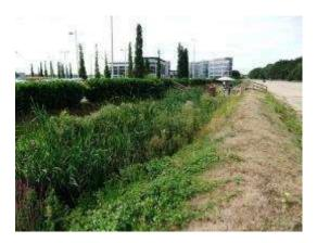
Fig 5.53 - Wide drainage channel, constructed c.2005 alongside the eastern edge of the Railway Straight, as part of the flood alleviation measures for the northern end of the Brooklands site.
