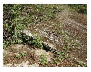
Fig 5.115 - Areas of collapse and undermining to the top edge of the banked track.
