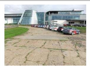
Fig 5.44 - Various degrees of surface degradation to the track, including some tarmac surfacing and modern patch repairs.
