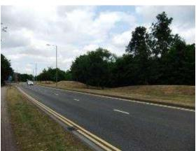
Fig 5.92 - Bunds and tree planting along the western edge of the characterisation area, preventing unauthorised vehicular access from Sopwith Drive.
