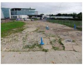
Fig 5.45 – Significant surface degradation to the northern end of the 'Sahara Straight'. Inappropriate replacement concrete bay in the foreground.
