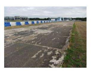
Fig 5.46 - Remains of tarmac top coat to surface of 'Sahara Straight' and erosion to track bays along their outer edges. (Radley House Partnership)
