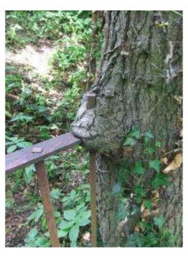
Fig 5.80 - Sections of railings being consumed by the growth of the trees along the support banking.
