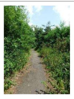
Fig 5.84 - Encroaching vegetation along the sides of the Aerodrome Road, leading to the loss of the edges and making its alignment difficult to distinguish.
