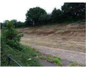
Fig 5.100 - Encroaching vegetation to the lower and top edges of the rack track, and further scars of inappropriate interventions by utility companies along the lower edge.
