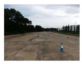
Fig 5.41 - Further surface degradation, patch repairs and scars of previous uses on the track towards the southern end of the Railway Straight.
