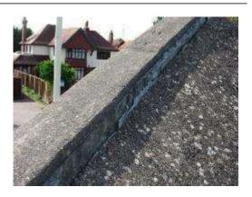
Fig 5.106 - Failed mastic type sealant at the abutment of the former track edge and the retaining wall to Barnes Wallis Drive, clear evidence of movement in the track surface.
