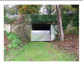
Fig 5.8 – Southern entrance to the Competitors' Tunnel, structural movement evident on left hand side.
