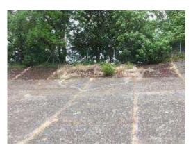
Fig 5.7– Vegetation and weed growth becoming established to areas of track degradation.
