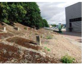
Fig 5.112 - Gravel has been laid over a geotextile membrane in the location of the lost inner edge to the track.
