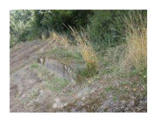
Fig 5.98 - Concrete base, associated with World War 2 defence measures, cast through the top edge of the race track.
