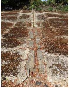
Fig 5.114 - Scar running though track, indicative of a former fence line with post holes to the left of the main groove cast through the surface.
