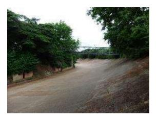
Fig 5.12 – Members' Banking to the north-east side of Members' Hill. Air raid shelters built into the Hill and the scar in the track surface showing the late-twentieth century repairs in the location of the former hangar.
