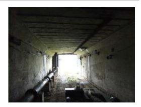
Fig 5.9 – World War 2 alterations to interior of the Competitors' Tunnel evident to the lowering and reinforcement of the ceiling. (Radley House Partnership)
