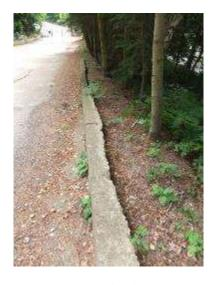
Fig 5.19 – Low-level in-situ cast concrete kerbing to the south-western edge of Dunlop's Delight.
