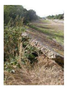
Fig 5.101 - Significant areas of undermining to the top edge of the race track as a result of burrowing animals. (Radley House Partnership)
