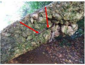
Fig 5.74 - Evidence of bar reinforcement to the now unsupported top of the banked track (southern end).
