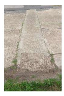
Fig 5.47 - Line of services cut through the track surface at 'Howe's Corner', inappropriately filled and finished.
