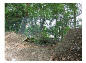
Fig 5.6 – Partial collapse and undermining to the top edge of the race track
