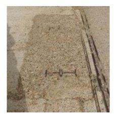
Fig 5.39- Remains of a Bellman hangar T184, including the metal channels for the sliding doors and metal columns now cut off flush with the raised concrete floor (laid over the former race track).
