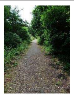
Fig 5.83 - Areas of wear and surface degradation to the tarmac finish, exposing the aggregate to the hardcore base below.
