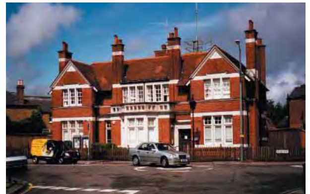
The Police Station (1901) is an important building with a robust architectural character.
