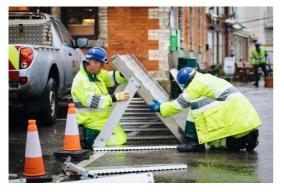
Temporary barriers can be deployed when flooding is forecast and are removed once flooding has subsided. They require 24/7 security, maintenance and seepage pumping, so they are only appropriate as a short-term measure whilst floods are ongoing. They are appropriate for use in minor to moderate flooding, which happens more frequently than extreme or severe floods. The barriers are not suitable for severe flooding where water levels will outflank the barriers or exceed their height.
