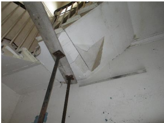
Left: August 2014 the main cantilever staircase in the Home of Compassion propped up Right: The staircase in 2016 following repairs and stabilisation
